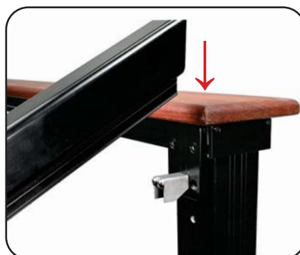
(8) Set Top Rail in Place Place top rail onto RCB to ensure the cut and fit are correct.
