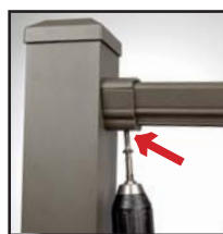
Fasten top rail to bracket
