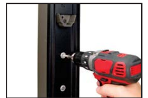
Fasten Threaded Connectors
