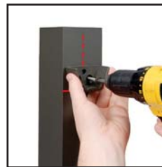
Center bracket and attach to post
