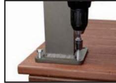
Fasten Post to Deck Surface
