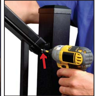
(b) Anchor Bracket w/ pivot screw
