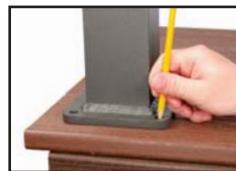
Mark and Pre-drill Holes
