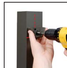
Center bracket and attach to post
