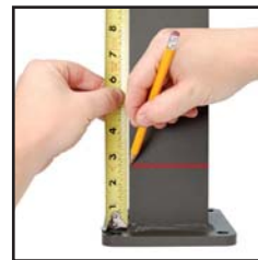
Measure up 2-1/2" from top of base plate
