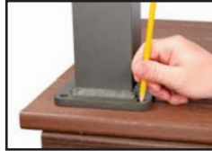
Mark and Pre-drill Holes
