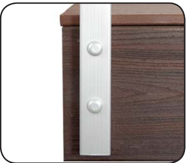
Step 10: Finished fascia mount post installed.
