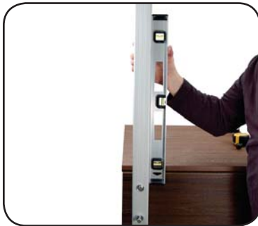
Step 9: Plumb post, adjust as needed. Tighten fasteners and ensure proper engagement into blocking.
