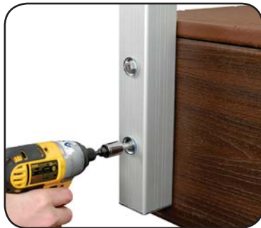
Step 8: Install cup washer under head of each fastener and drive fastener loosely into blocking.
