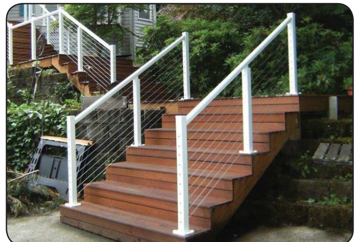
Series 100 Rail - Terminating Into End Posts
