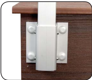
Finished fascia mount bracket with post installed.
