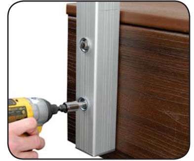
Step 7: Confirm location of fascia post. (Max. post spacing of 50" on center) Mark holes, remove post and drill pilot holes to accept 3/8" lag or carriage bolt.
